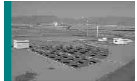
Fig 11: View of the photovoltaic field
