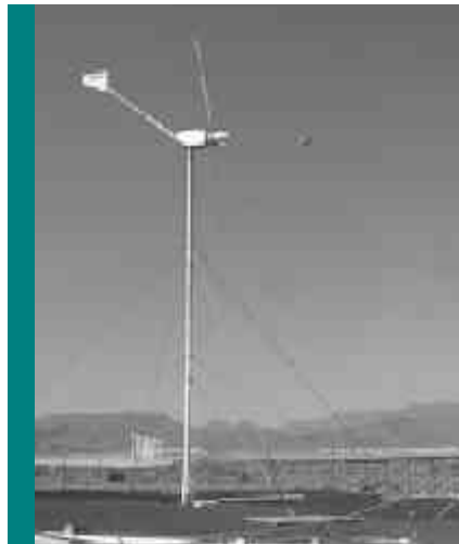
Fig 9: Windturbine -a commercial one-
