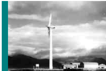
Fig 15: View of the technical installations
