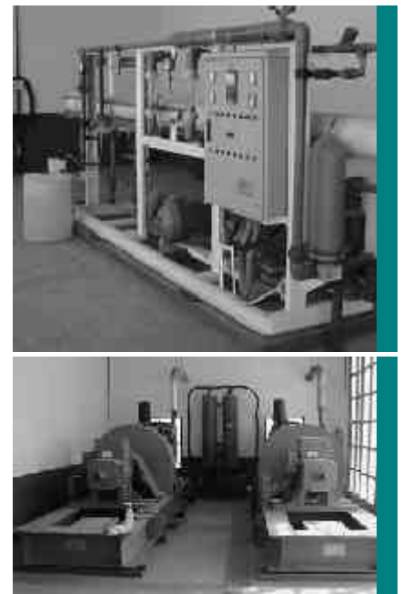
Fig 17: View of the diesel system (2 x 60 KW)
