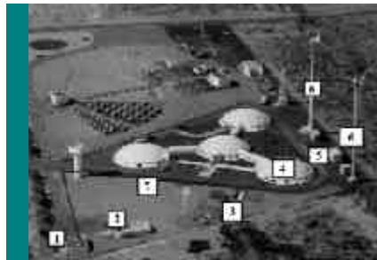
Fig 1: General view of the installations. (1) Pumping Station. (2) Product water tank. (3) Brackish water tanks. (4) Desalination dome. (5) Flywheel building. (6) Wind Turbines. (7) Feed water pipe circuit
